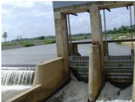
Photo32: Derivation gate for providing water
